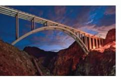
A dramatic new concrete arch joins the setting of the historic Hoover Dam, spanning the Black Canyon between the States of Arizona and Nevada. The 1,900-foot-long Colorado River crossing is the centerpiece of the \$240 million, fourlane Hoover Dam Bypass Project, which included 3.5 miles of new approaches on both sides of the river and seven other bridges.
