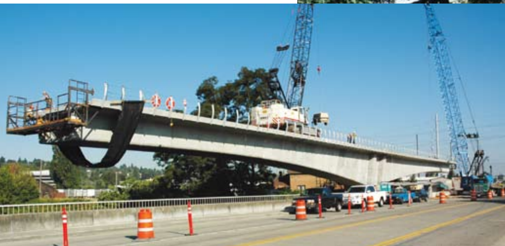
Construction of the 350-ft span over the Duwamish River. Photo: IBT.
