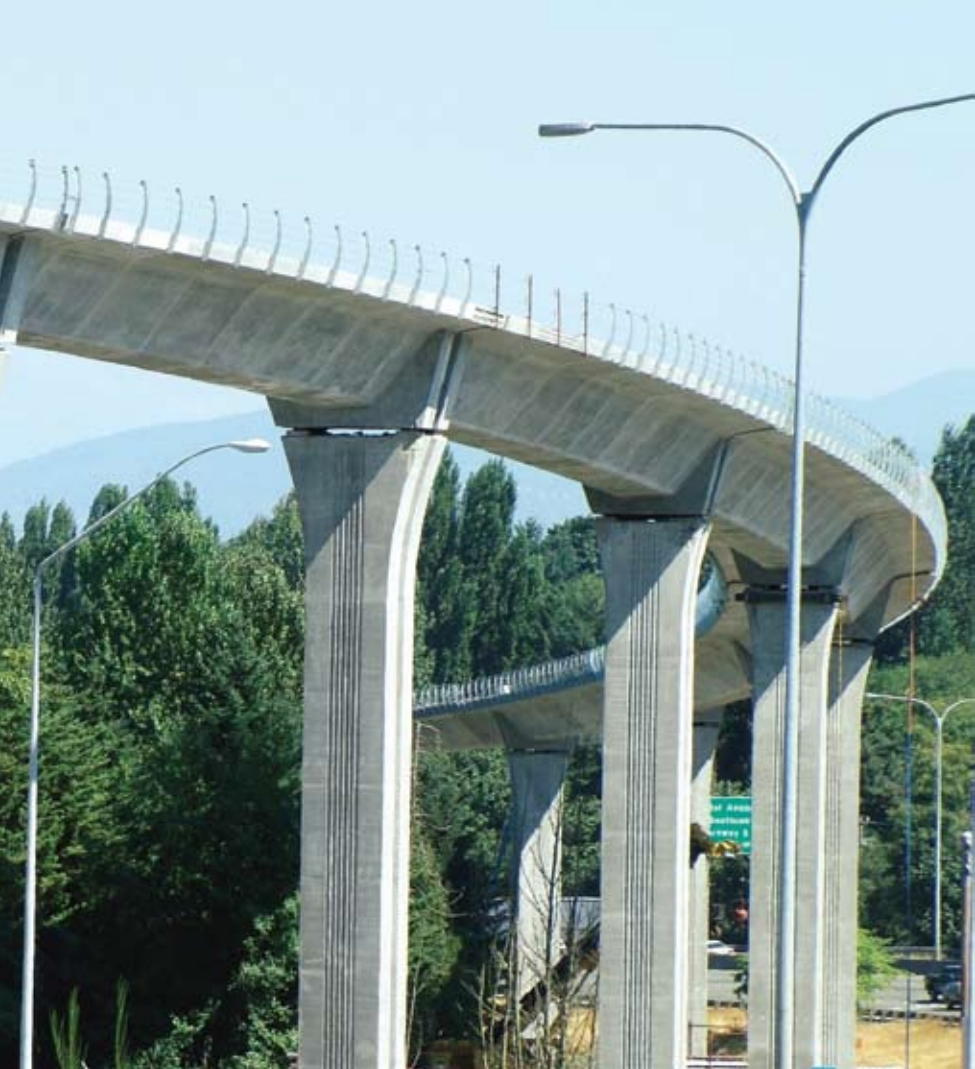
The winding, twisting bridge includes super elevations as well as horizontal and vertical curves, all compensated for in the casting of the segments. Photo: Hatch Mott MacDonald.
