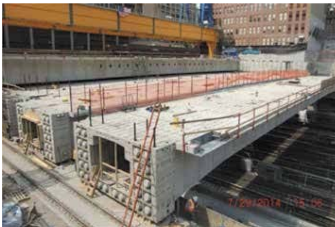
Fig. 6—Post-tensioning on face of pier segments.
