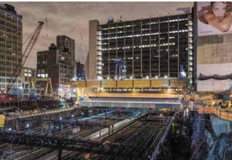
Fig. 3—View of jobsite.
