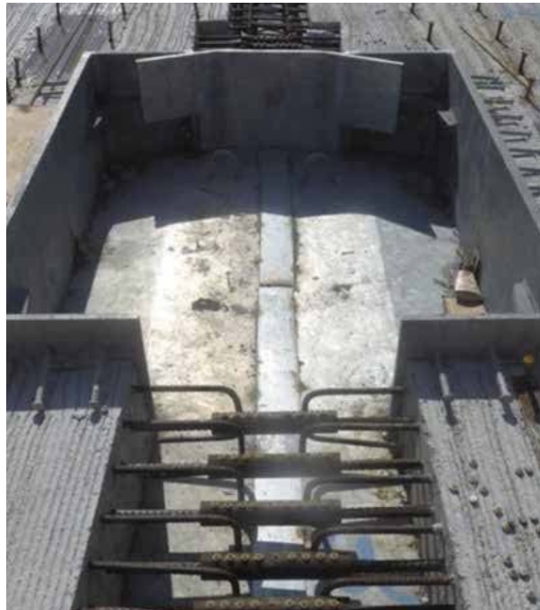
Fig. 9—Column openings.
