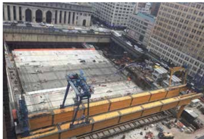
Fig. 7—Cast-in-place operations.
