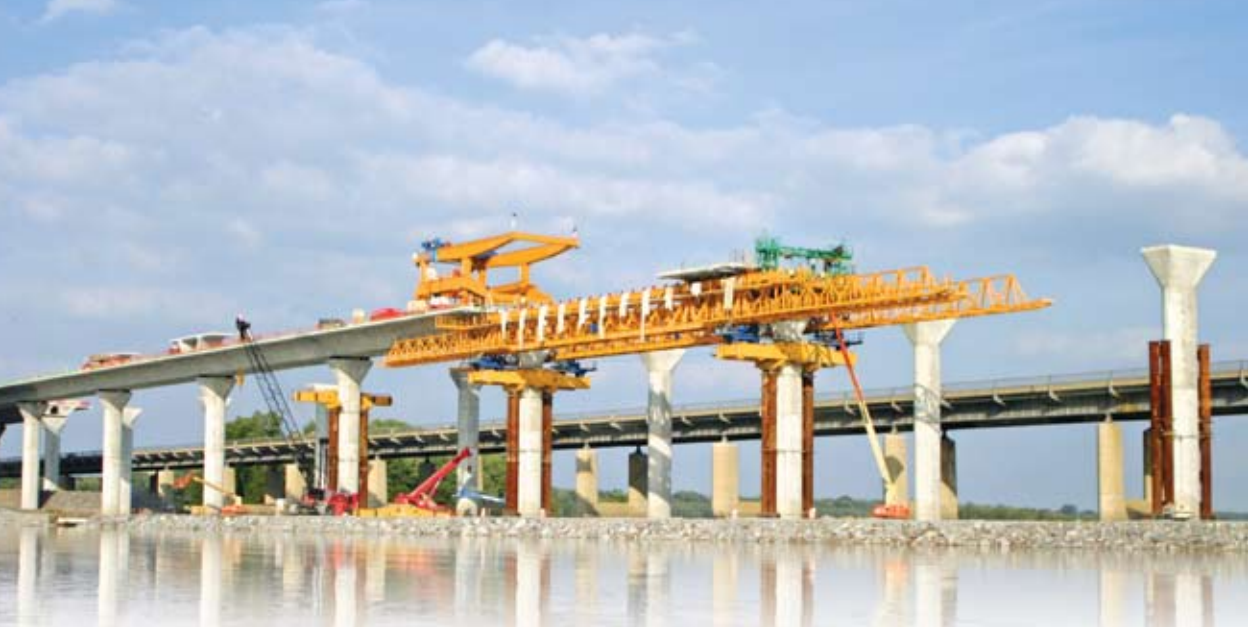
An underslung erection truss was used with the span-by-span method of construction.
