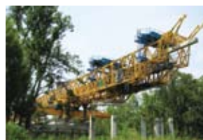
The pile is loaded into the lead with an attachment for the hammer clamped to its top. The lead then rotates the pile into a vertical position for driving.
