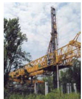
The pile is loaded into the lead with an attachment for the hammer clamped to its top. The lead then rotates the pile into a vertical position for driving.
