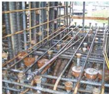
*Diaphragm cage and column reinforcement.*
