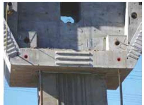
*Completed diaphragm and monolithic pier connection.*
