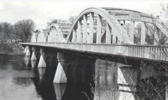
Early photo of the four consecutive concrete tied arch spans of the Covered Bridge in Norridgewock, Maine, constructed in 1928. Photo: Maine Department of Transportation.
