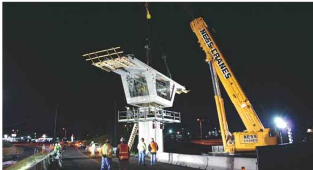
1061-FT-LONG, FOUR-SPAN, PRECAST CONCRETE SEGMENTAL BOX-GIRDER BRIDGE / WASHINGTON STATE DEPARTMENT OF TRANSPORTATION, OWNER
