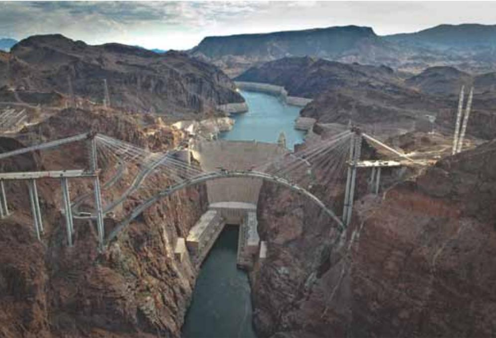
McNary Bergeron provided construction engineering for the cast-in-place arch structure and temporary stay-cable system used to support the Hoover Dam Bypass Colorado River Bridge. It was one of the first high-profile projects for the company, which was founded in 2003. All photos: McNary Bergeron & Associates Inc.
