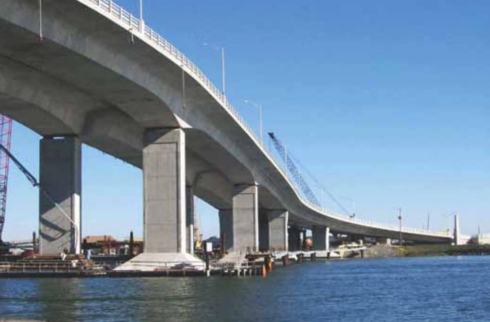
Speed of construction was a key reason that McNary Bergeron helped create the all-precast concrete design for the Route 36 Highlands Bridge over the Shrewsbury River in Monmouth County, N.J. Each of the twin bridges were cast and erected in a construction season, providing access year round while construction continued.
