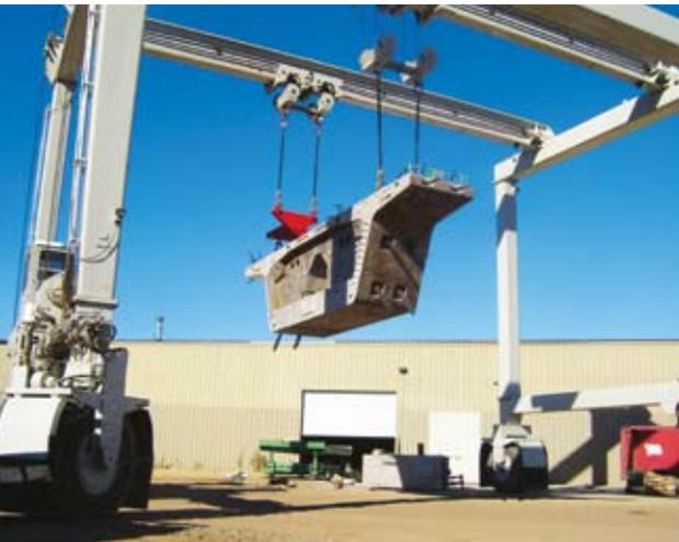
With the casting of this pier segment on October 18, 2007, Minnesota's first precast concrete segmental bridge gets underway. Photo: Mn/DOT.
