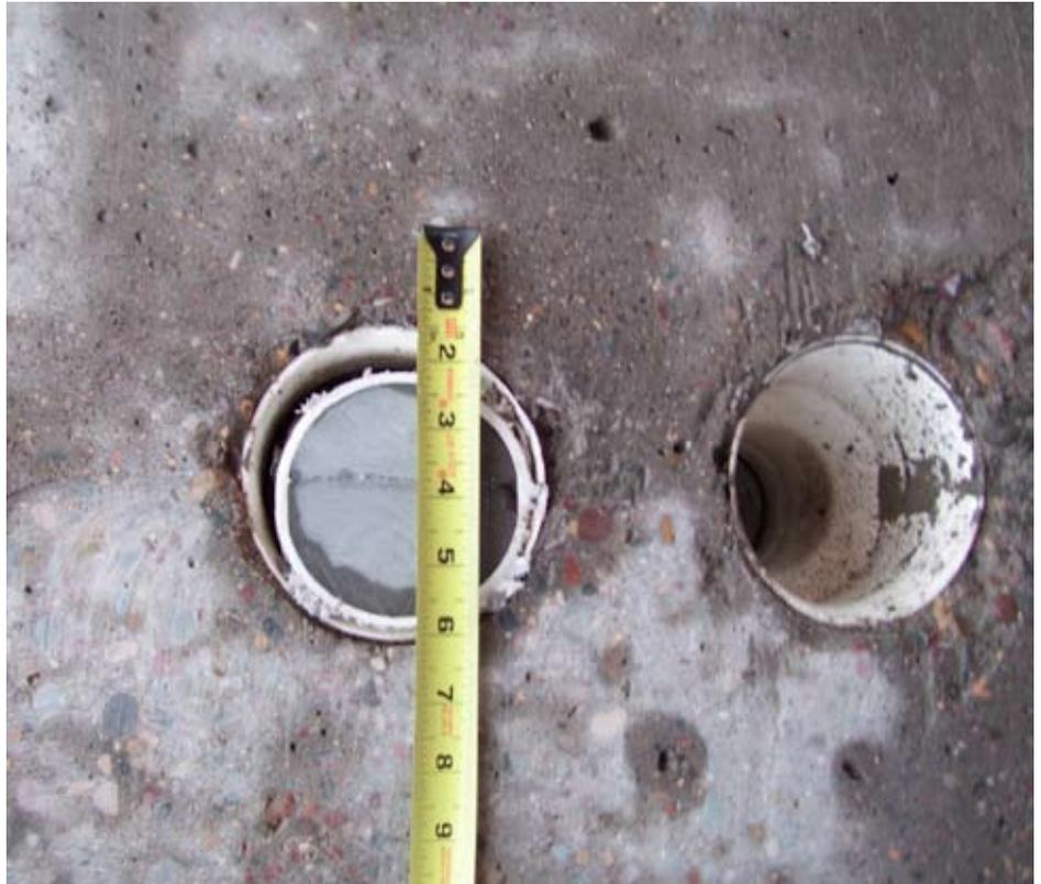
The void area around the duct coupler raised concerns where chlorides could potentially collect in the top slab. The duct couplers were tested, but not used within any of the Crosstown segmental bridges. Photo: Mn/DOT.
