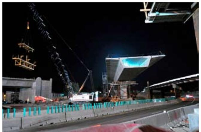
Short-term closures occurred at night to allow for safe erection over traveled ways. Photos: © FIGG.
